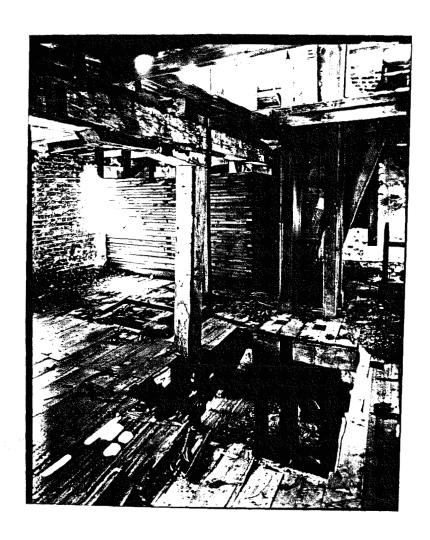
PLATE 11: DUCK CREEK MILL, INTERIOR SECOND FLOOR OF SOUTHEAST CORNERS OF PHASE II AND III STRUCTURES. FRAMING IS PRIMARILY OF REUSED TIMBERS REWORKED AT VARIOUS TIMES THROUGHOUT ITS HISTORY
