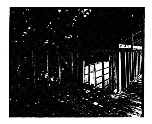
PLATE 12: DUCK CREEK MILL, INTERIOR ATTIC LEVEL OF PHASE I STRUCTURE. NOTE THE THREE SETS OF RAFTER BLADES IN CENTER BACKGROUND AND THE USE OF COLLAR BEAMS WITH HALF-DOVETAIL AND HALF-LAPPED JOINTS. IN THE LEFT FOREGROUND NOTE THE HEAD ARRANGEMENT FOR THE EXTANT BANK OF GRAIN ELEVATORS.
