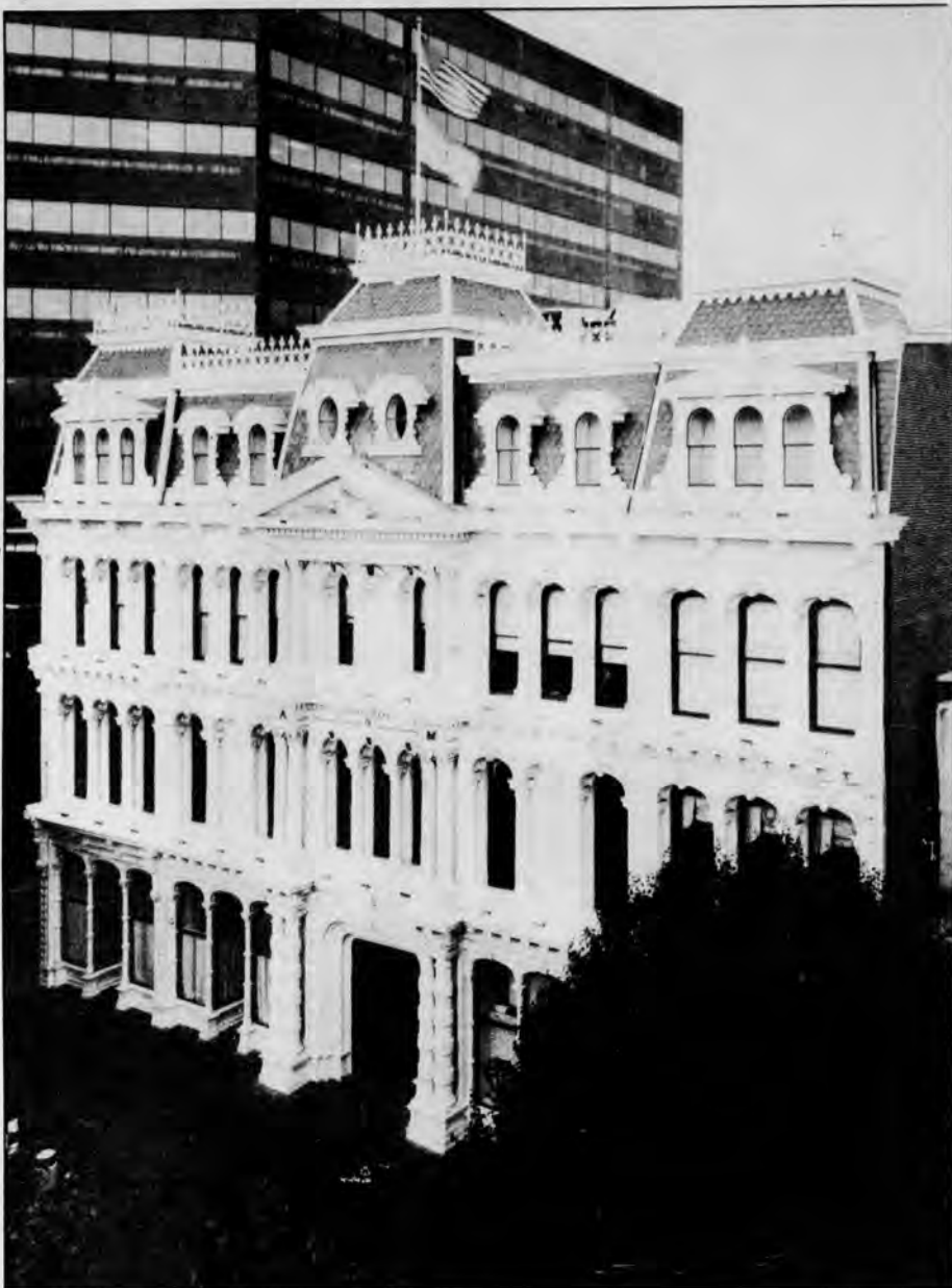
The Grand Opera House proudly shows off the restoration which brought it national honors. Wrote the Advisory Council on Historic Preservation, the Grand restoration is "one of the finest examples of cast iron cleaning, casting and repair which we have documented."
