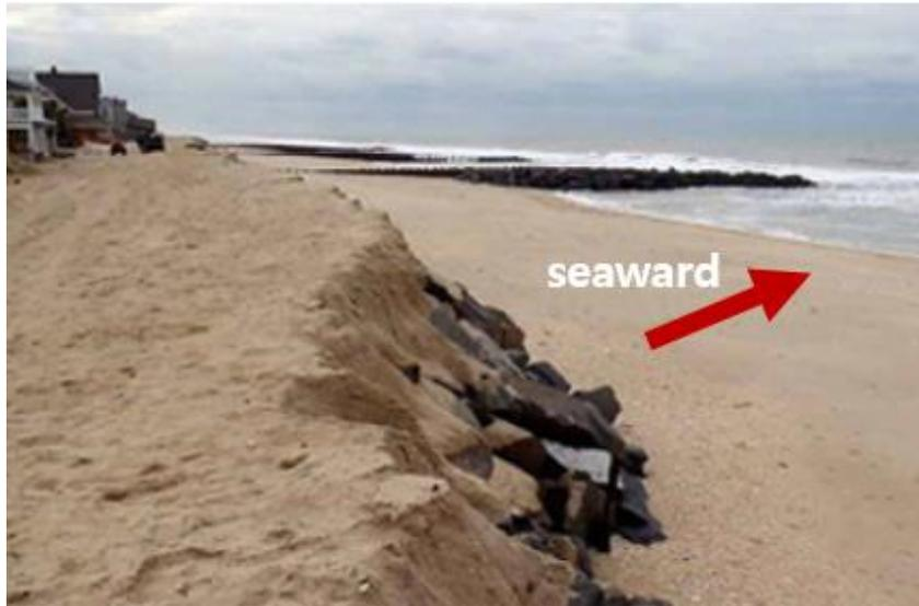
Figure 1.1: Partially exposed relic rock seawall after Hurricane Sandy (Irish et al. 2013)
