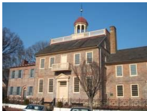
New Castle Court House, Delaware Street, New Castle, New Castle County
