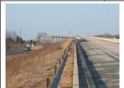
Reedy Point Bridge, S. Reedy Point Road, Route 9, Delaware City, New Castle County
