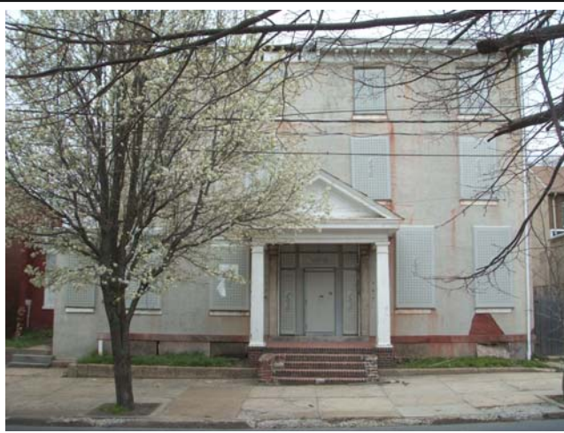
Elwood Garrett House, N. Washington Street, Wilmington, New Castle County
