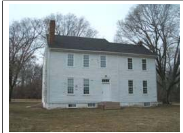
Brecknock Park, Old Camden Road, Alternate Route 13, Camden, Kent County
