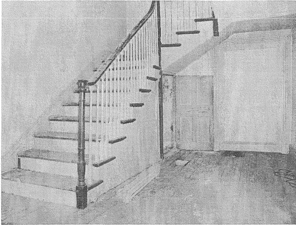
K-0000-9: Interior center hall stairway, cellar entrance and sealed rear door detail. Also note paneling, newel post and balustrade detail. Regular width floorboards laid east/west.
