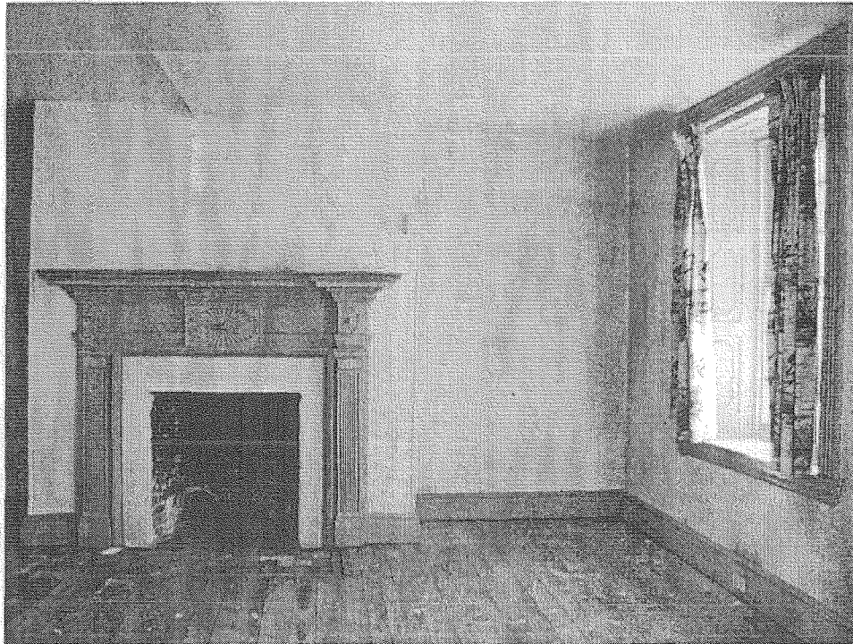
K-0000-11: Interior, stone block, first floor south parlor. Fireplace mantle decoration and west window paneling detail.
