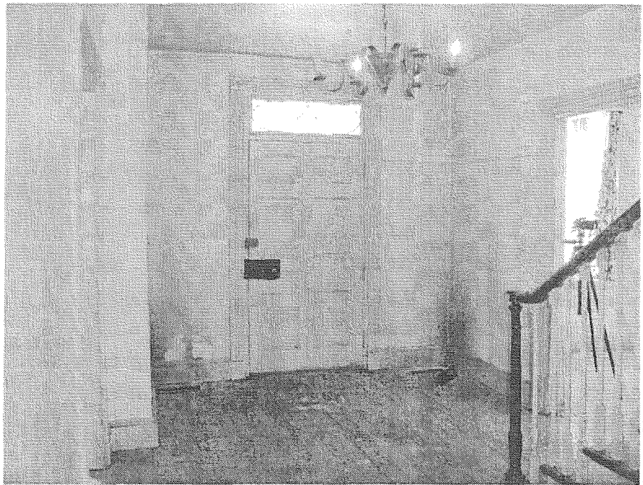
Figure 5. Interior, center hall perspective of main block. Front door details include deep reeded moulding, bulls-eye corner blocks, and a fanlight. The floorboards in the room run east to west.
