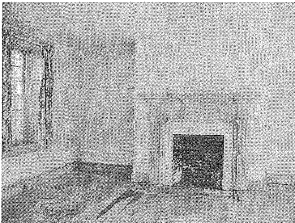
K-0000-12: Interior, stone block, first floor south parlor. View of east window paneling detail and south wall fireplace and elaborate reeded mantle detail.
