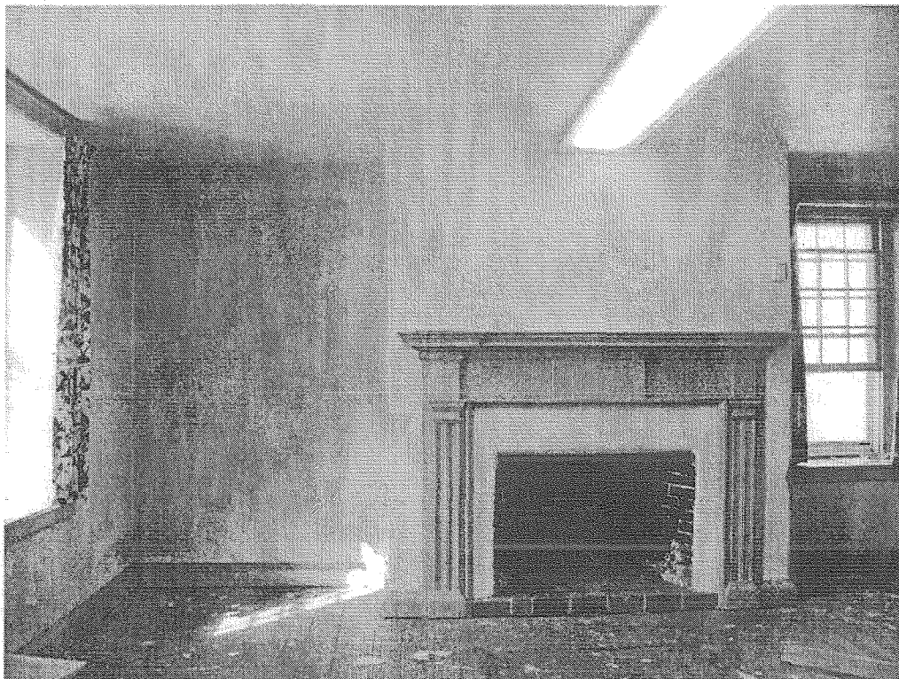
K-0000-10: Interior, stone block, north parlor first floor. North wall fireplace, mantle and sealed window detail. Regular width floorboards laid north/south.
