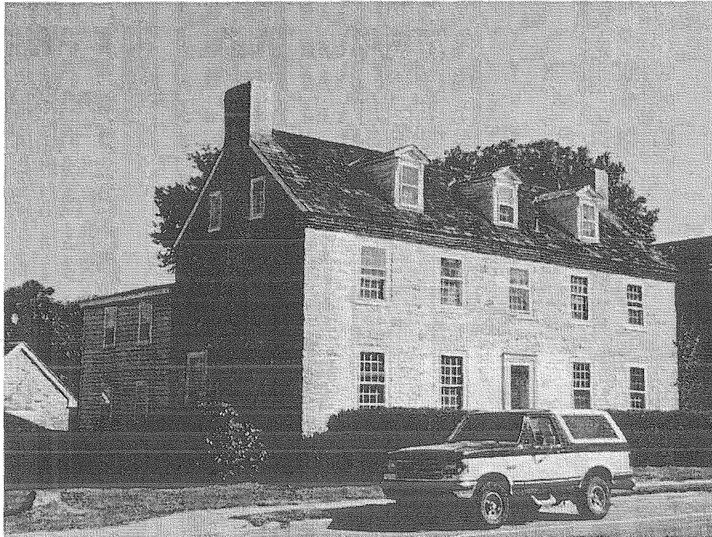
Figure 3: Perspective of west and north elevations showing the Period I stone block, Period II frame shed addition, and stone outbuilding.
