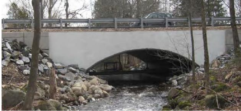
Figure 4. Completed Neal Bridge. Photo 1. Completed Neal Bridge. Reprinted from Project case studies for IBRC and IBRD Programs , D. Paterson et al., 2012, FHWA report, p.858. Unpublished internal document of FHWA.
