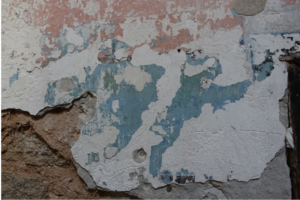
Figure 75 Self-excavation: the ruining process has made the paint peel in Eastern State Penitentiary, revealing different layers of paint colors that existed at different times, but are now showcased together. In this way, the different paint colors highlight different layers of history and how they coexist today. Photo by Natalie Wright. Eastern State Penitentiary, Philadelphia, PA.
