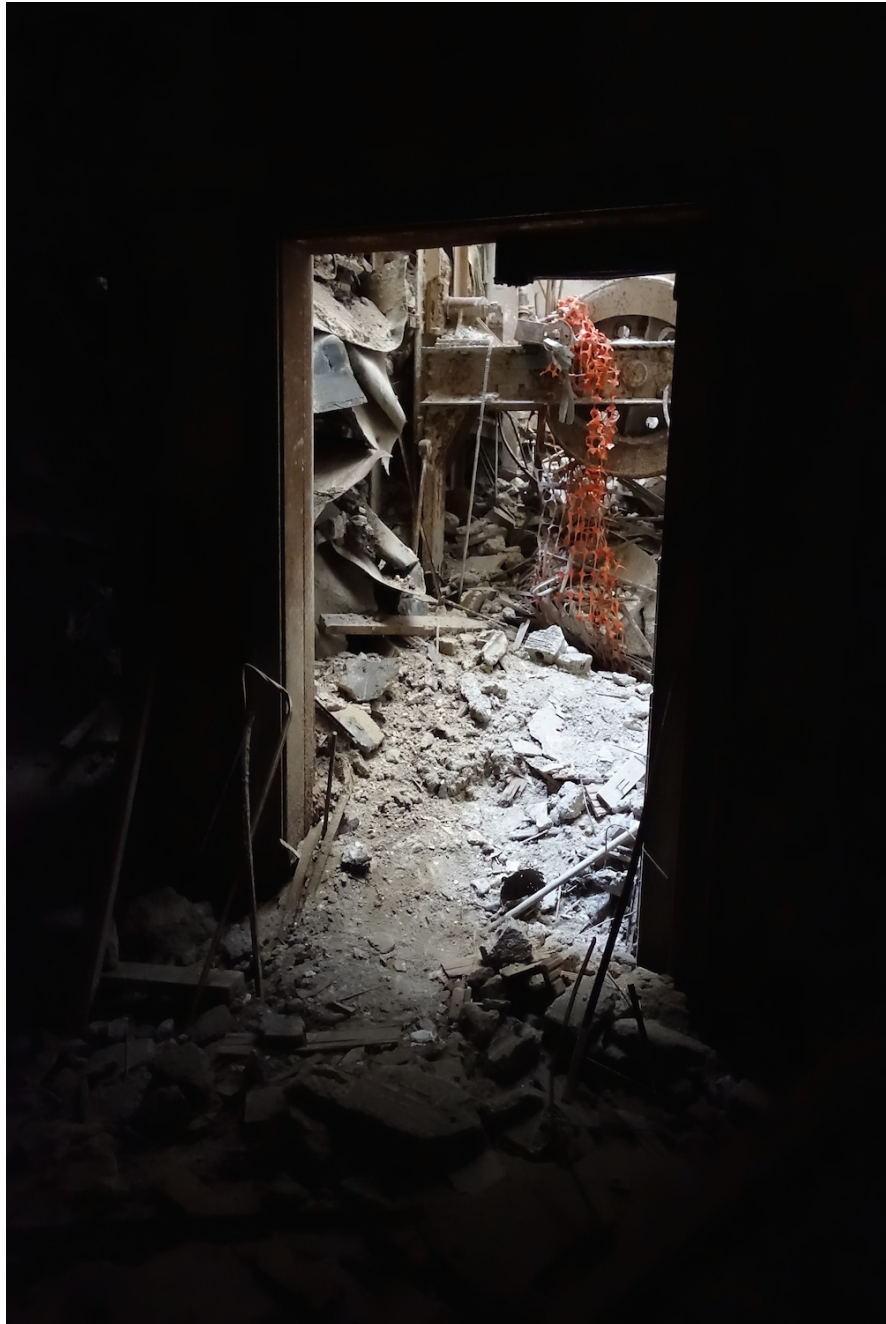
Figure 26 Natural light pours in from the elevator shaft to reveal debris that has come down from crumbling walls. Photo by Natalie Wright.
