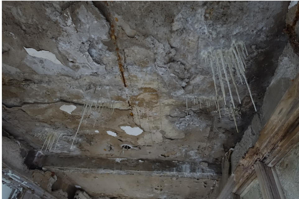
Figure 29 An otherworldly scene: Stalactites fall from the ceiling, as minerals from the concrete drip down over time. Photo by Natalie Wright.
