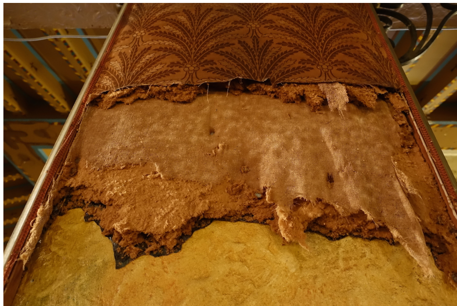
Figure 73 Self-excavation: the deterioration of upholstered walls in the Lansdowne theatre, revealing the layers beneath. Photo by Natalie Wright
