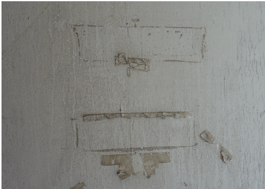
Figure 55 Material memories of objects: an example of tape witness marks, where the tape's glue has left a residue indicating where other objects, such as signs, may have been. Photo by Natalie Wright.
