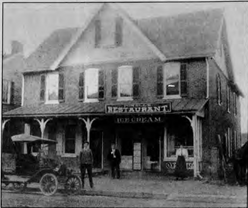
The site of the former Powell's Restaurant, shown in this early century photograph from the Newark Historical Society, is included in recent land sale.
