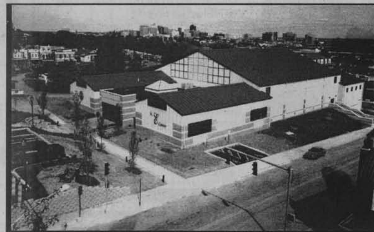
The St. E Center - St. Elizabeth High School's new 25,000 square foot academic and athletic facility was dedicated by Bishop Michael Saltarelli on Sept. 15, 2001.
