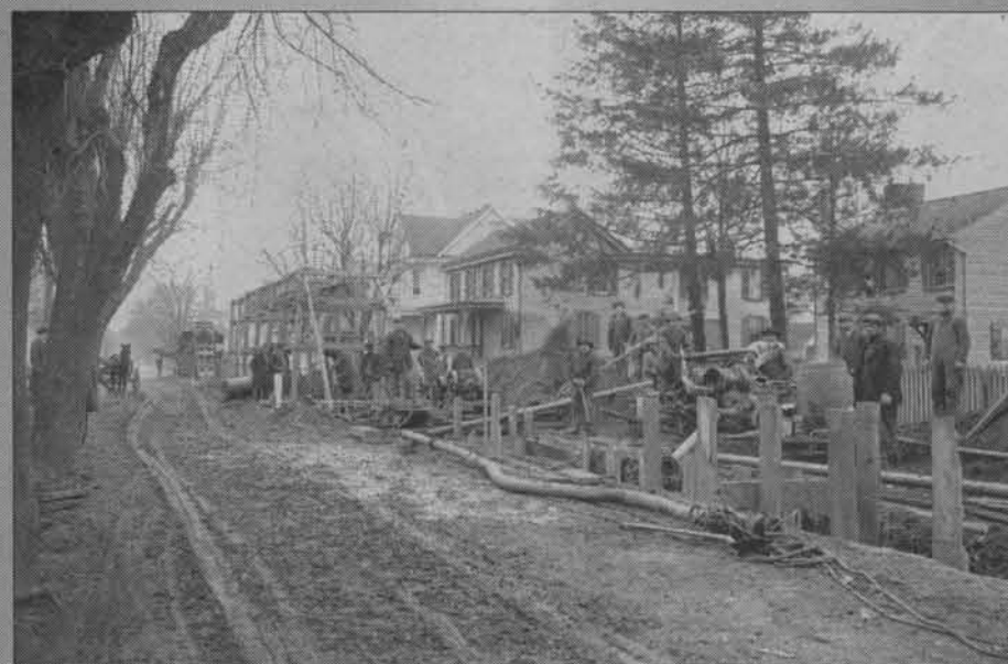
This week, "Out of the Attic" features a photograph of a Newark roadway, possibly Main Street, taken in the the 1890s or early 1900s, courtesy of the University of Delaware Archives. UD's Ian Janssen noted that the photo shows the dirt streets that existed in Newark in the early years of the 20th century. The installation of pipe work, shown here, was necessary prior to any street paving. "Out of the Attic" features historic photographs from Newark's history, recent and long ago. Readers who have a historic photo and would like to share it with other readers are invited to loan their photos for reprinting in this space. Special care will be taken. For information, call the Newark Post , weekdays, 8:30 a.m. to 5 p.m., at 737-0724.
